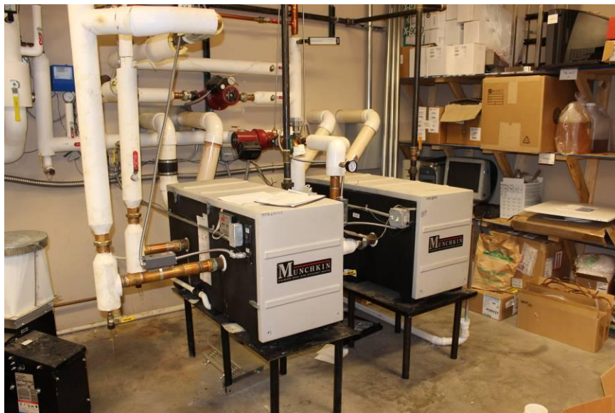
Sample view of mechanical boilers.
