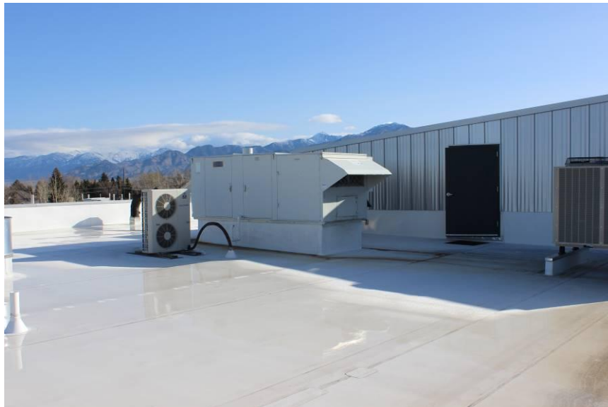
Sample view of roof and RTU HVAC.
