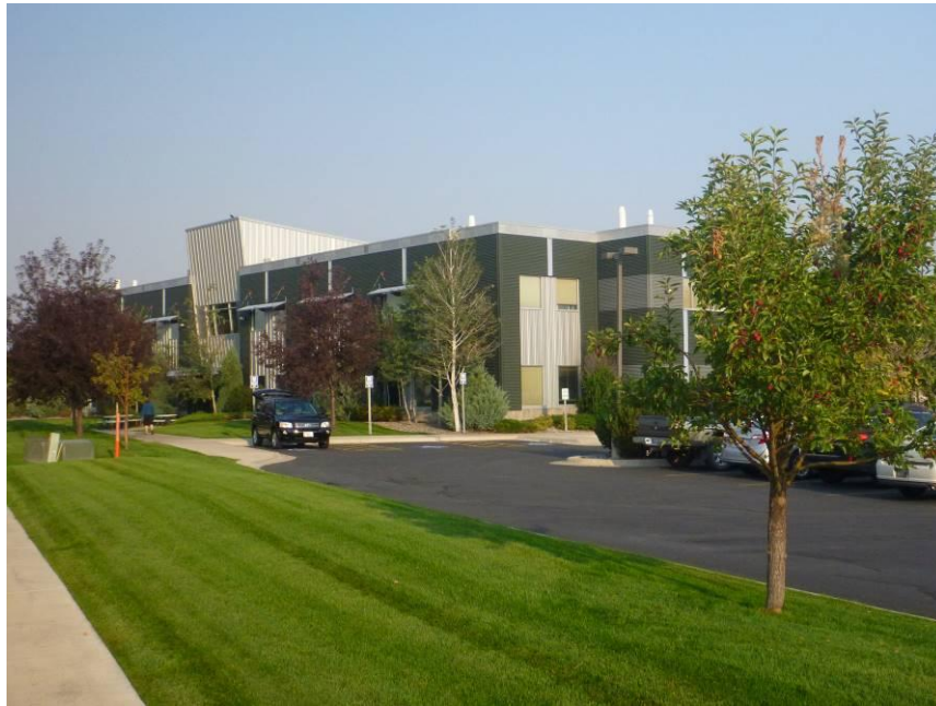
View of the front of the subject property. Photo taken on August 25, 2015 by Keith O'Reilly, MAI.
