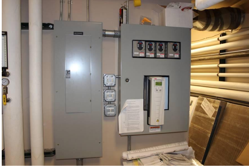
Sample view of electrical panels.
