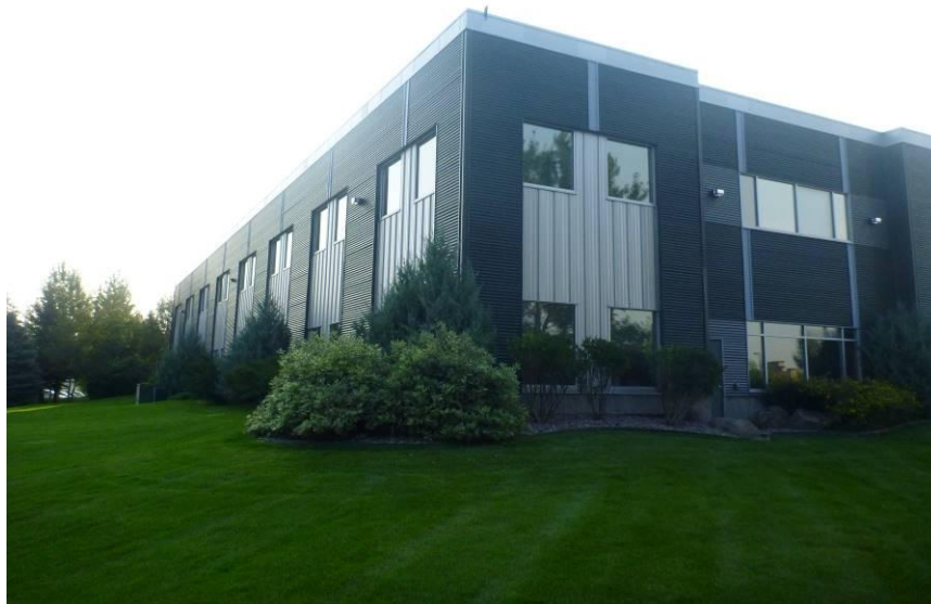
View of the north and west side of the subject property. Photo taken on August 25, 2015 by Keith O'Reilly, MAI.
