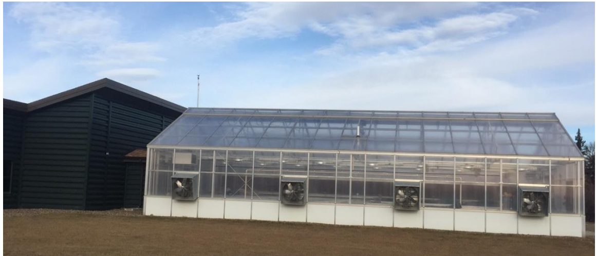
Eastern Agricultural Research Center greenhouse-headhouse new construction, 2010.
